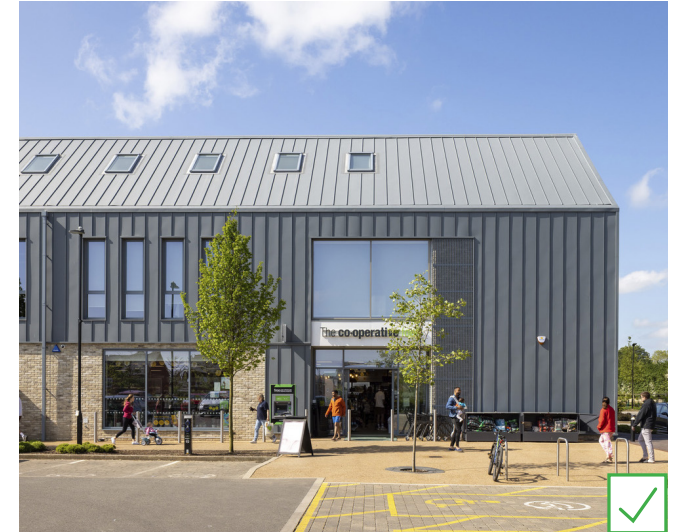
Clear signage and entrances designed as part of the elevation ensures user legibility
