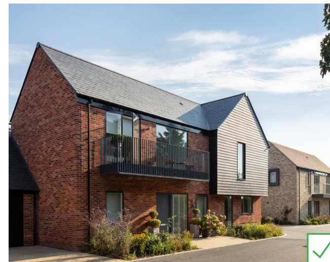
High-quality balconies designed to complement to overall composition of the elevation
