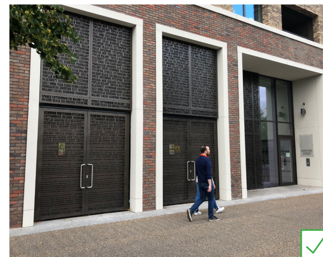
Refuse discretely incorporated into the building design
