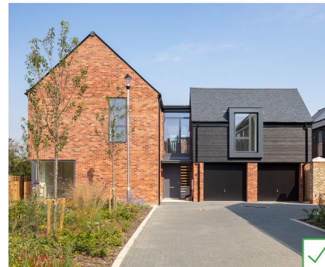
Dormer windows may also be intentionally offset if the overall composition is well considered
